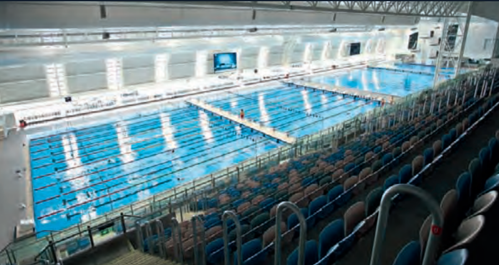
South Australian Center, Marion (Australia)
